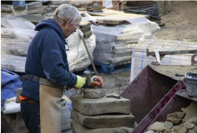
Previous page image: Stone Cutting at Abacus Stone Sales Top image: Stocks of reclaimed Yorkstone in the yard. Lower image: Cutting of reclaimed stone by hand to a specific dimension of 15cm. The width prepares it for the market and fits with current regulations.
